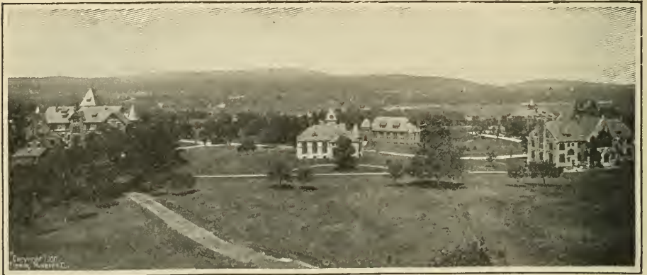
NORTHFIELD SEMINARY BUILDINGS AND CAMPUS FROM THE EAST.
